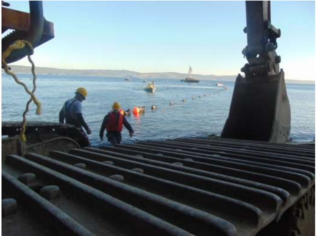
Floating part of the cable in the 2 nd landing point (Bell Island)
