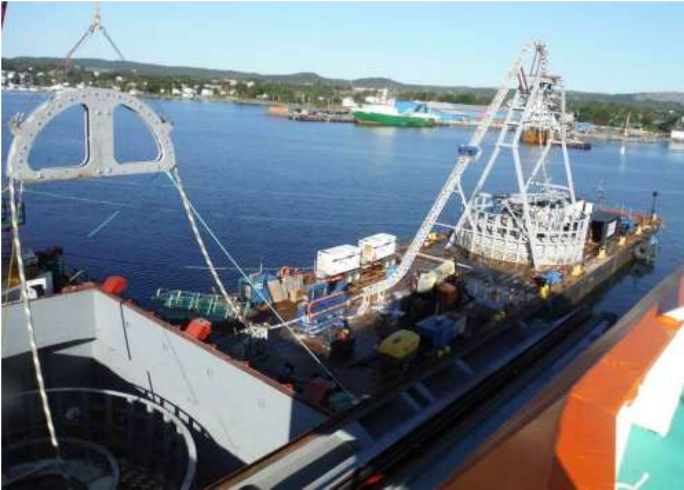
Loading between the transportation vessel and the installation barge
