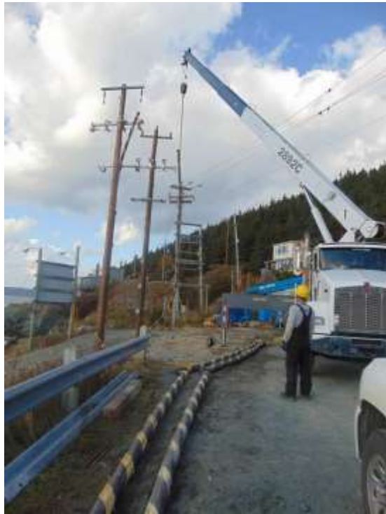
Lifting the cable in the termination pole.
